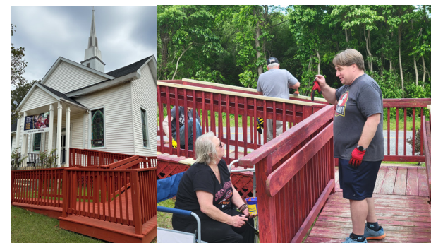
Volunteers repair ramp at St. UMC.
