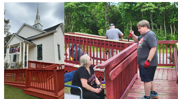
Volunteers repair ramp at St. UMC.
