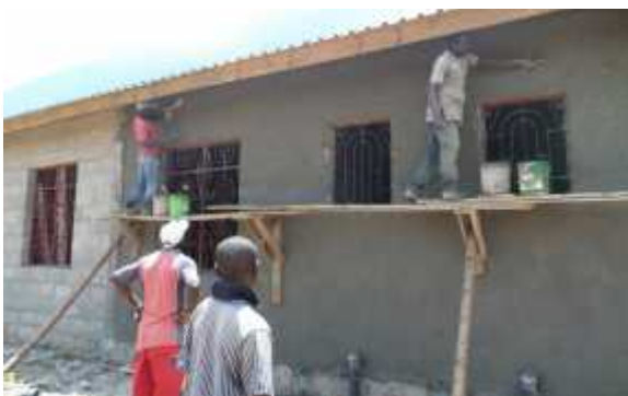
Guest House works in Dar Es Salaam
