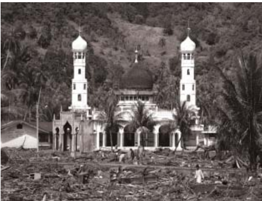
A Muslim Mosque stands relatively unscathed amongst a sea of debris and destruction in Banda Aceh. However, the mosque did sustain extensive water damage inside [UMNS photo]
